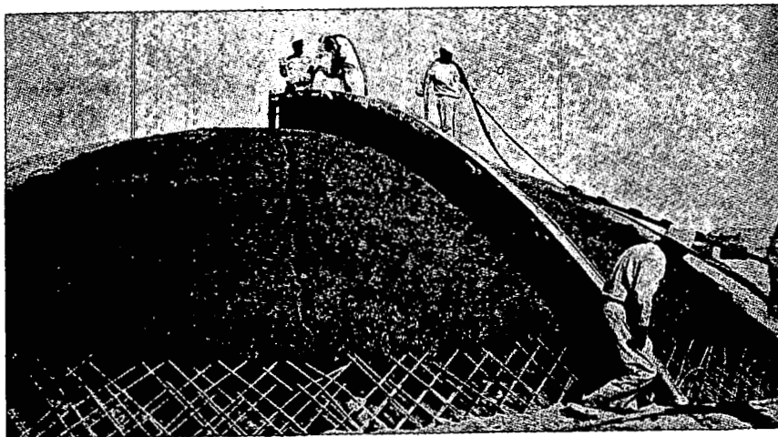
Fig. 8—Shotcreting of earth-berm form for responding concrete dome.
